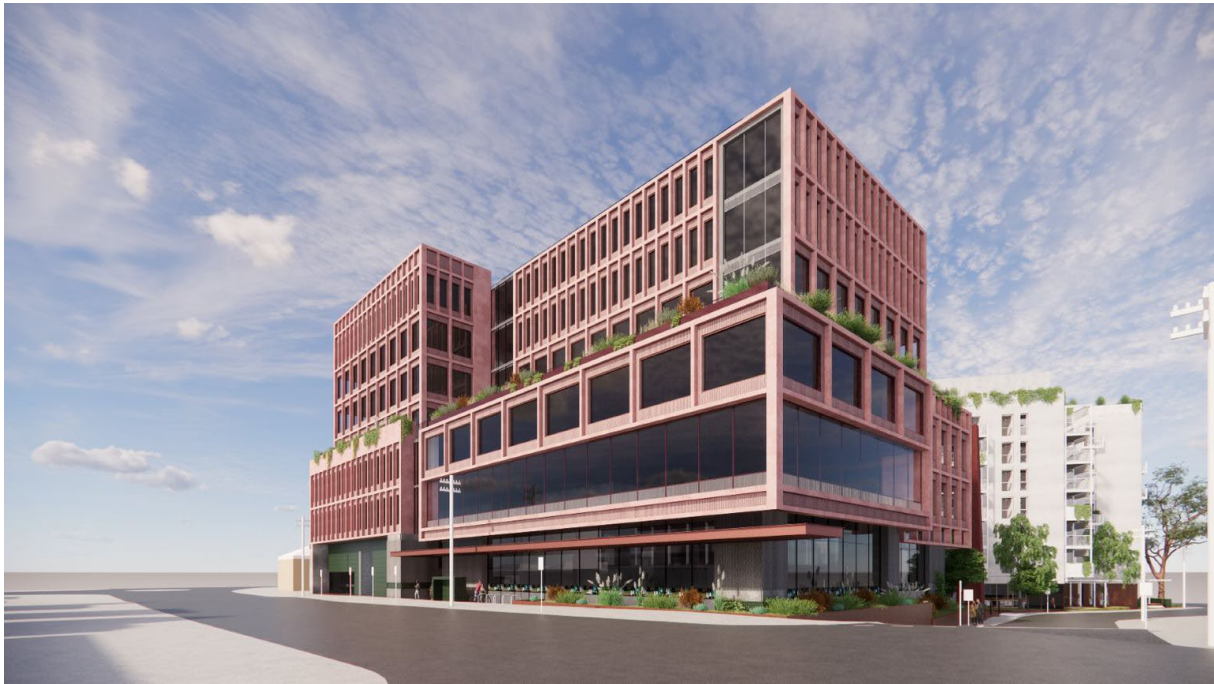
Figure 8 Alternate plan render from corner of Humffray Street South and Porter Street
