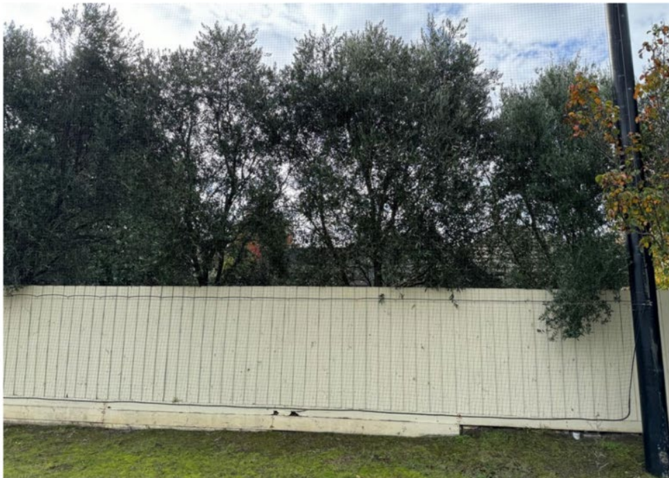
Photo of existing interface condition from with subject site
